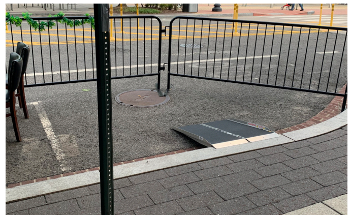
TEMPORARY ADA RAMP
